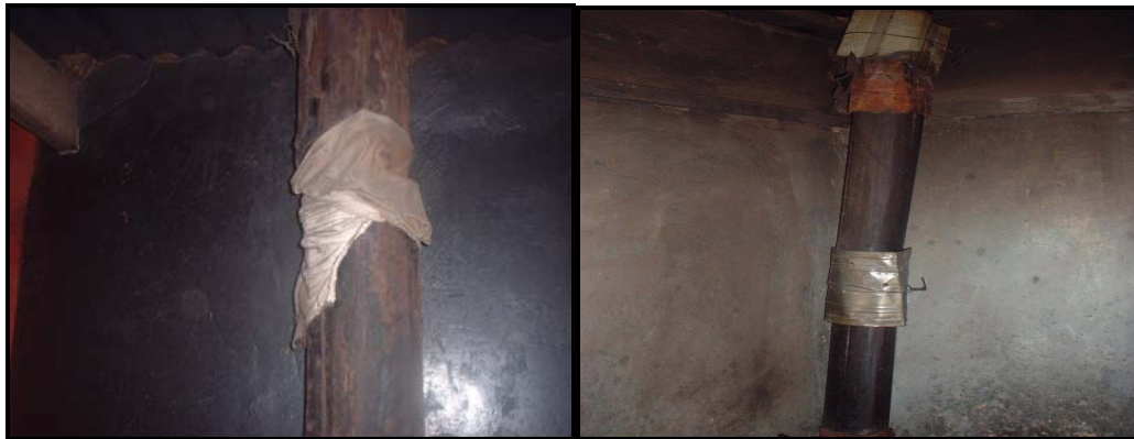
Figure 3 Methods of sealing chimneys
